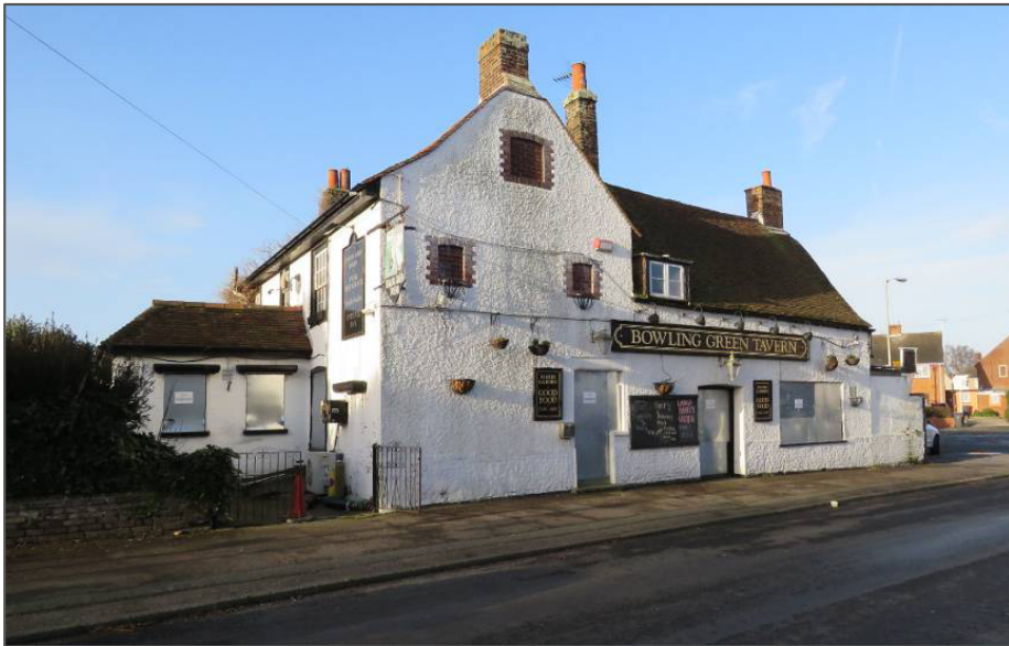
EXISTING EXTERNALS TO PUB
